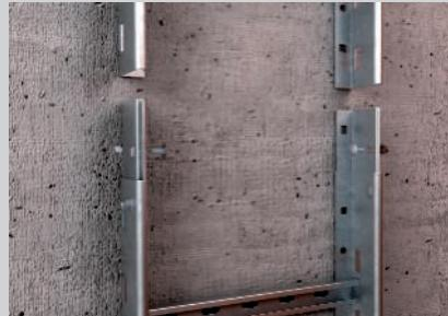
Joint connection with screwed-on connector.
