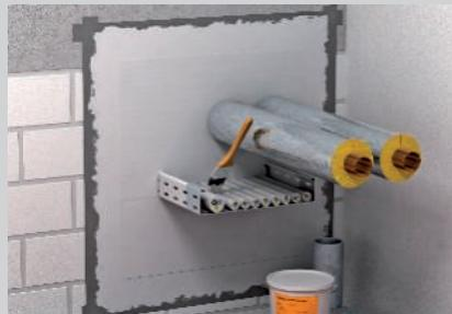
Apply the final coating to the surface and the installations.
