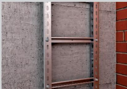
Direct mounting of the rising section on solid walls.
