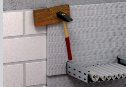
The plates can be inserted carefully with a hammer and board.
