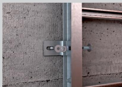
Mounting with screwed-on fastening brackets.
