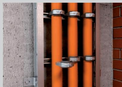
Cable installation with clamp clips on the rungs of the vertical ladder.
